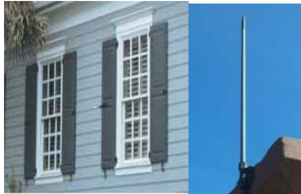
shutters and lightning rod
